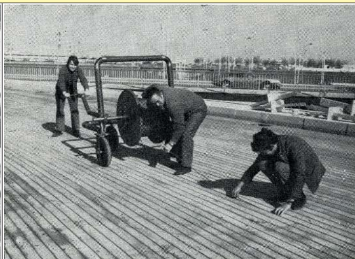
1968 Installation of the heating web on an access ramp to a bus parking platform, Orly airport near Paris (Electric floor heating, by Robert Félix, 1971, Ultimheat Museum*)
